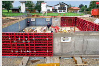
Wall Formwork
