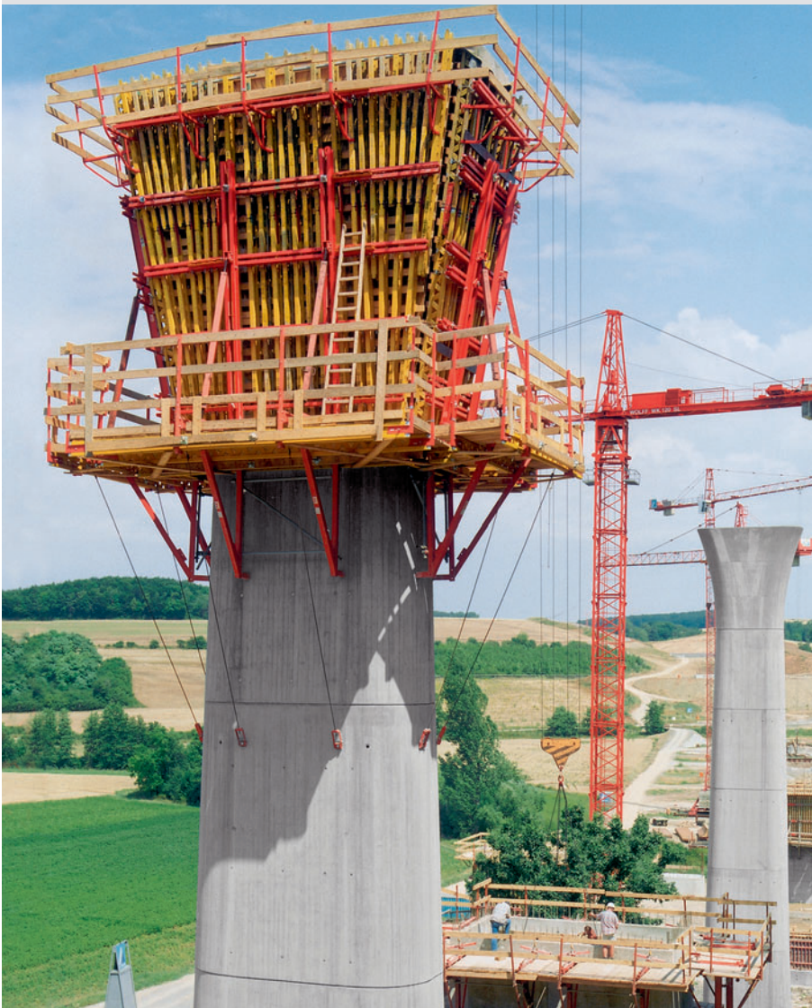
Pier head formwork with climbing scaffold and concreting platforms ready for casting.
