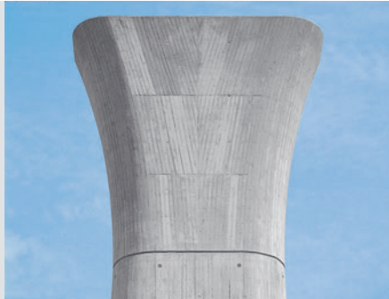
Exact and with the required board structure – one of altogether 16 pier heads after completion.
